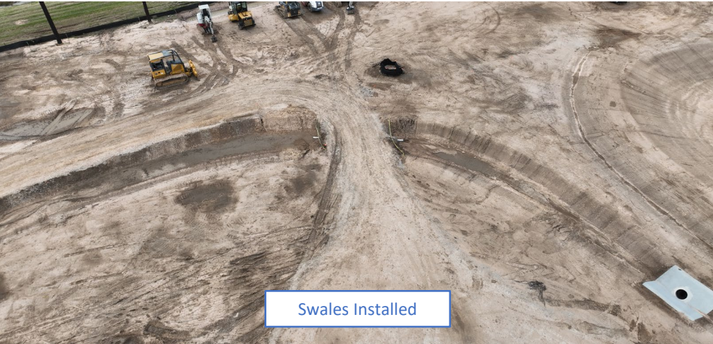
Detention Pond Grading Complete
