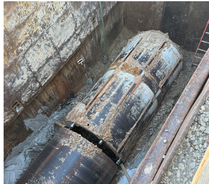
Contract 65 – West Little York Tunnel Machine Retrieval
