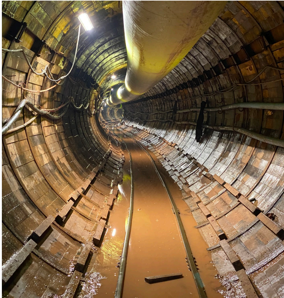
A1-A2 - Little York Tunnel
