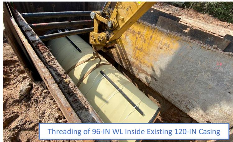
Threading of 96-IN WL Inside Existing 120-IN Casing
