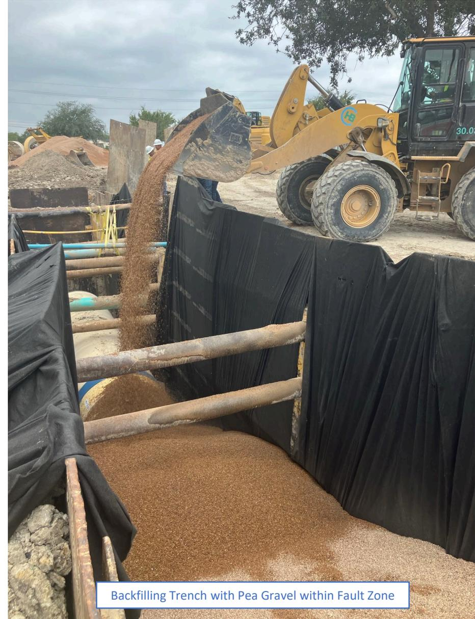
Backfilling Trench with Pea Gravel within Fault Zone
