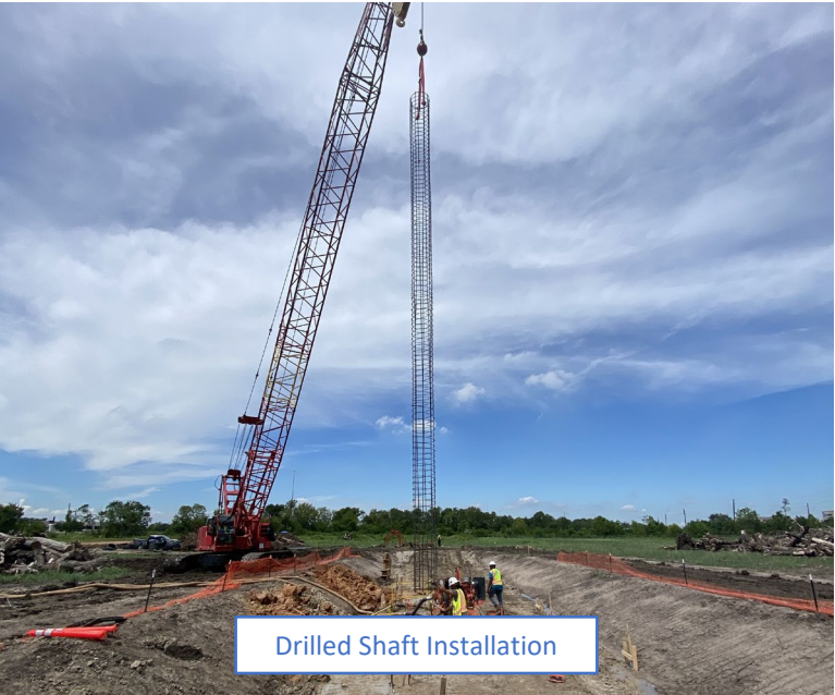
Drilled Shaft Installation
