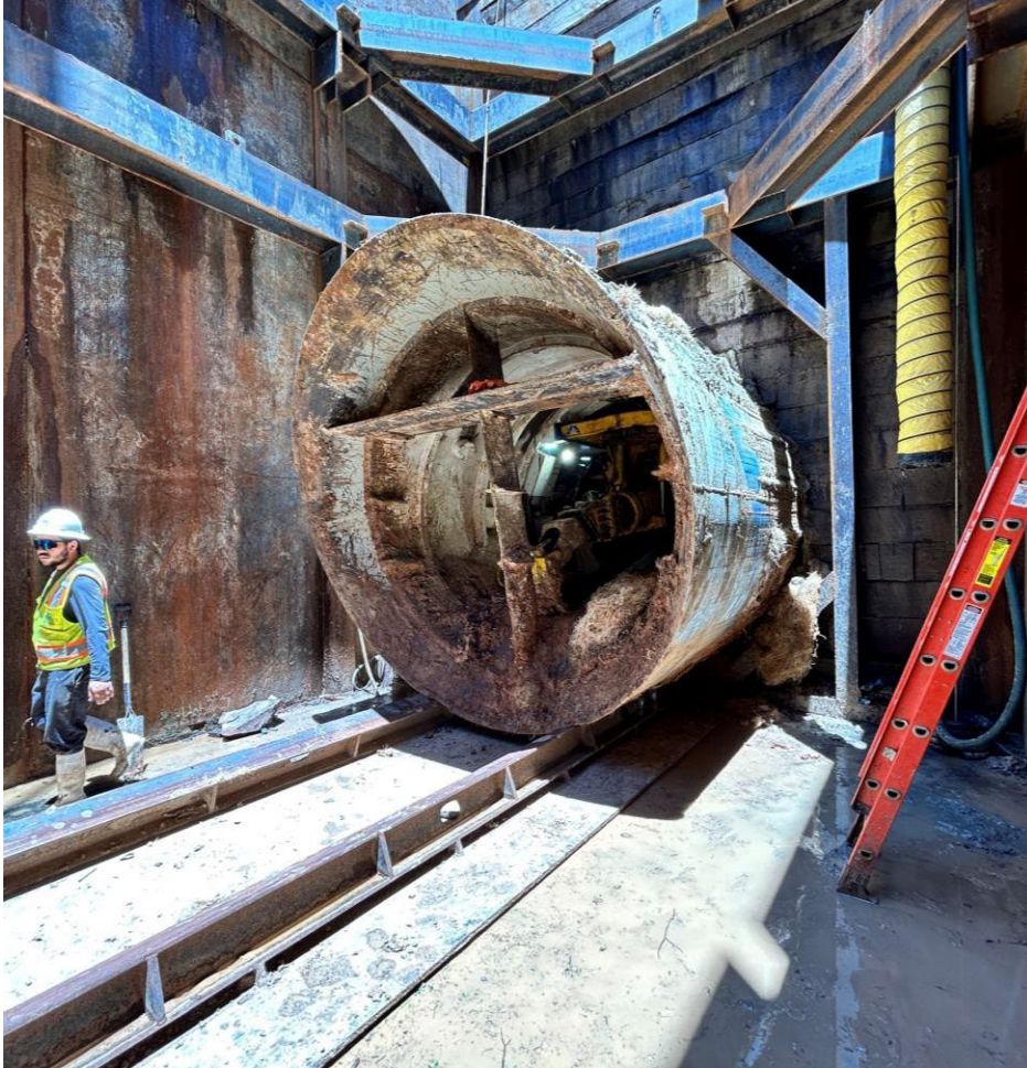
Segment A1/A2 – Mesa Rd. Tunnel
