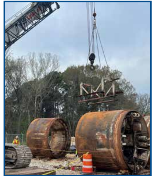
B3 - Reach 4 – TBM Retrieval (March 2024).
