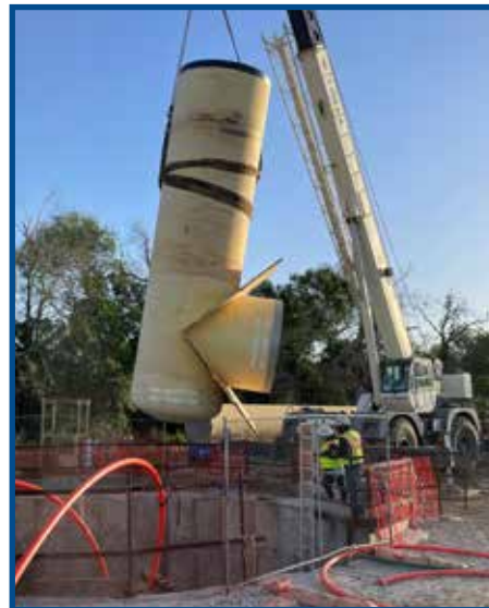
C1 - Installing Bear Creek Waterline 2.0 (March 2024).
