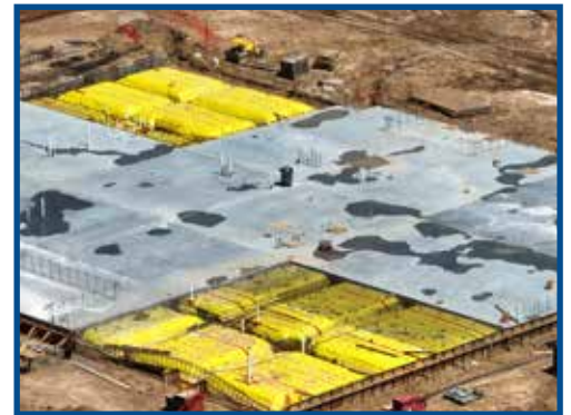
CPS - Operations Building Slab (March 2024).
