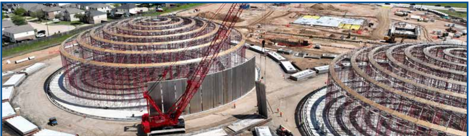
CPS - GST 1 Wall Panel Erection (March 2024).
