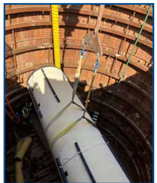
B1-B2 - Lowering Pipe to Thread 290 Tunnel (March 2024).
