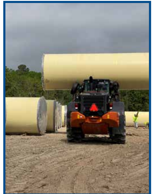
A1-A2 - Storage of 96-IN Waterline Pipe (March 2024).
