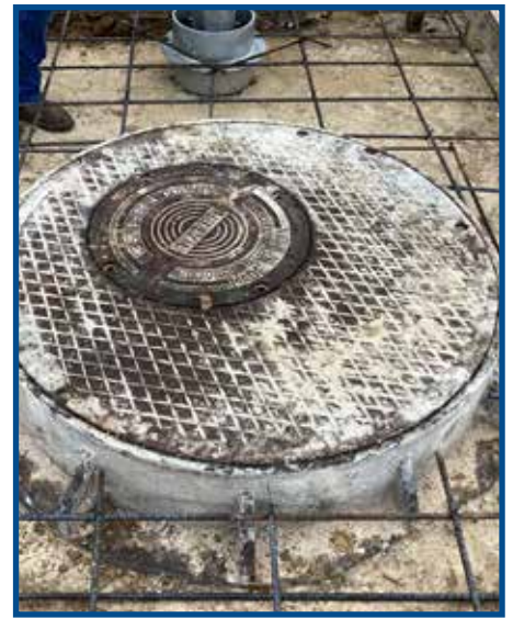
C2 - Framing and Rebar Installation at Manholes (March 2024).
