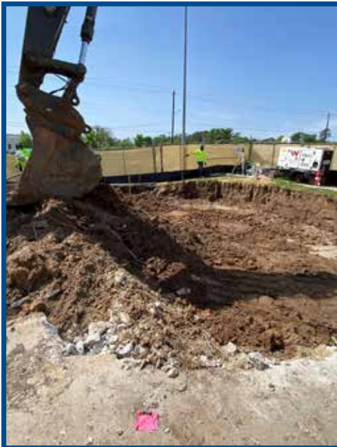
A1-A2 - Excavation of Homestead Rd. Receiving Shaft (March 2024).
