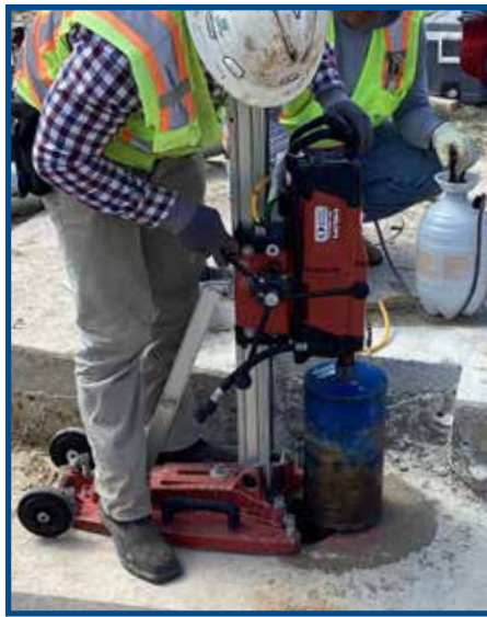
C2 - Coring ARV Outlet Piping (March 2024).
