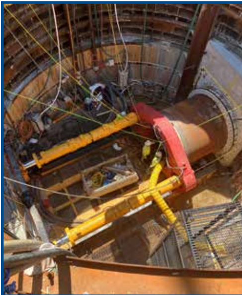
B1-B2 - Beltway 8 Connecting MTBM Utilities (March 2024).
