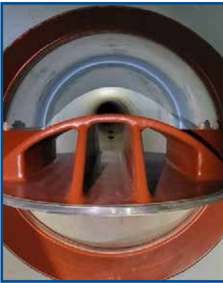
C2 - BFV Internal Restoration Complete (March 2024).
