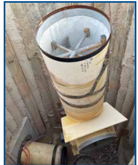
C1 - Installing Bear Creek Waterline (March 2024).
