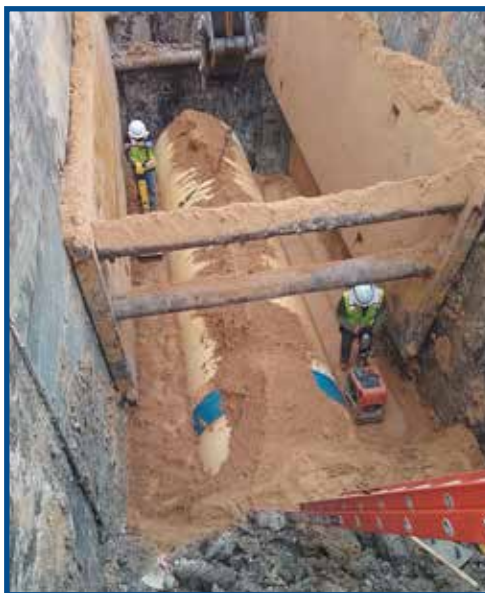
B1-B2 - Compacting Backfill on 96-IN Pipe East of Ella Blvd. (March 2024).
