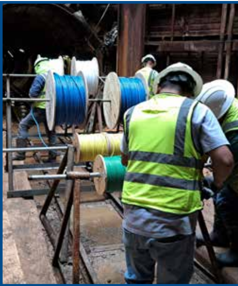
B3 – Cathodic Protection Installation (March 2024).
