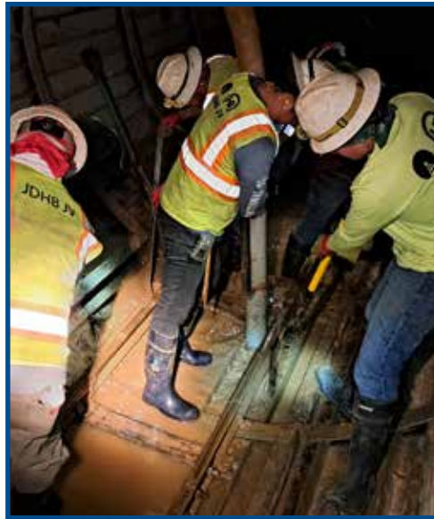
B3 – Reach 2 Tunnel Cleaning (March 2024).
