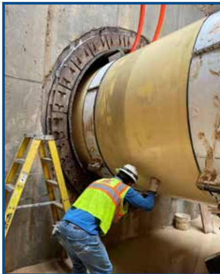
C1 - Bear Creek Waterline Installed (March 2024).
