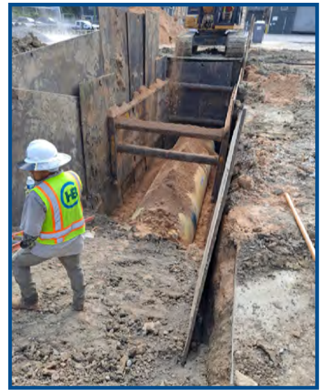
C2 waterline installation
