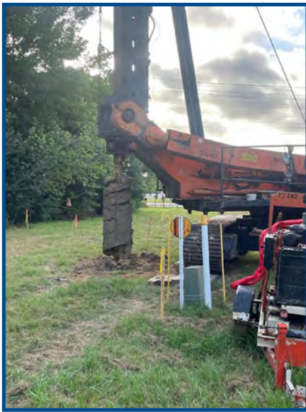
B3 removing deep anode well
