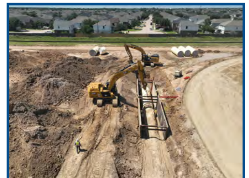
CPS Waterline installation
