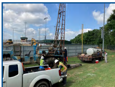
A1-A2 Performing Borings 2.0
