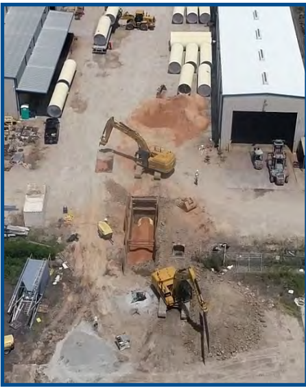
C2 open cut waterline
