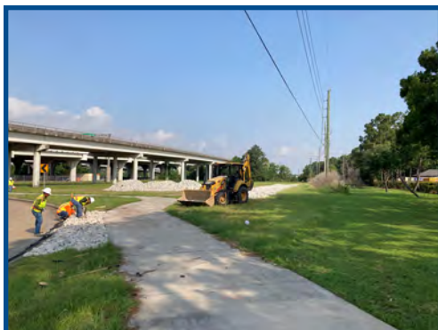
A1-A2 Installing construction entrances
