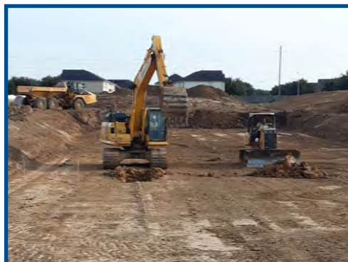
CPS Subgrade Preparation
