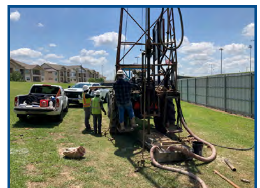
A1-A2 Performing Borings
