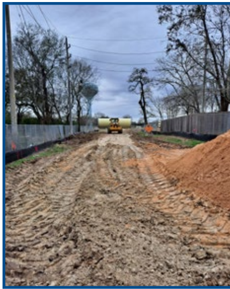
C2 Waterline corridor
