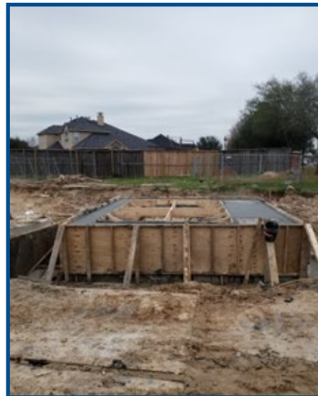
C1 Butterfly valve vault hatch poured
