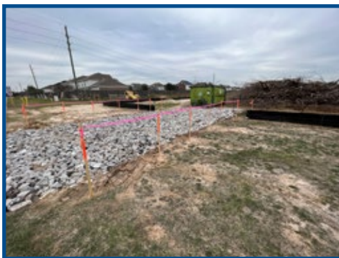
CPS Construction entrance and clearing operations
