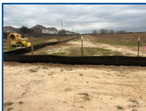
CPS Silt fence along existing pipeline corridor
