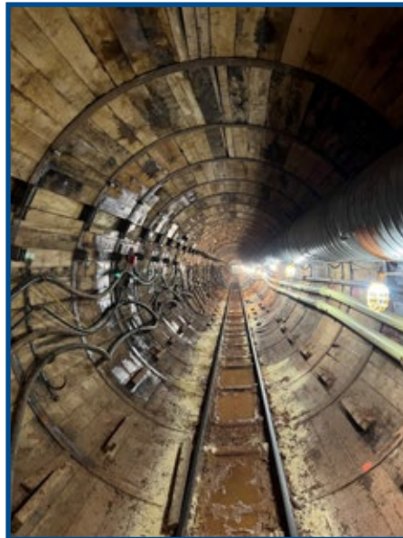
B1-B2 290 Tunnel looking West
