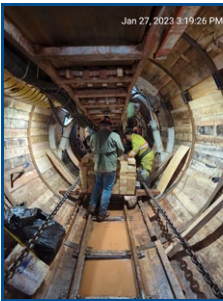
B3 Building Tunnel Rings
