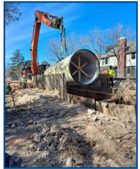
C2 Waterline open cut through Jamestown Colony
