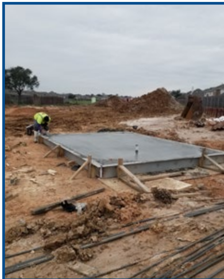
C1 Butterfly valve vault hatch poured
