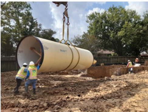
Handling Pipe within Concord Bridge
