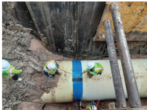
Installing Joint Wrappers
