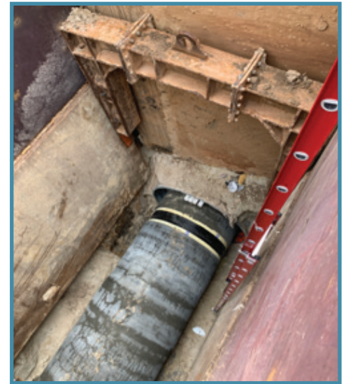
Installing 66-inch waterline in Tunnel
